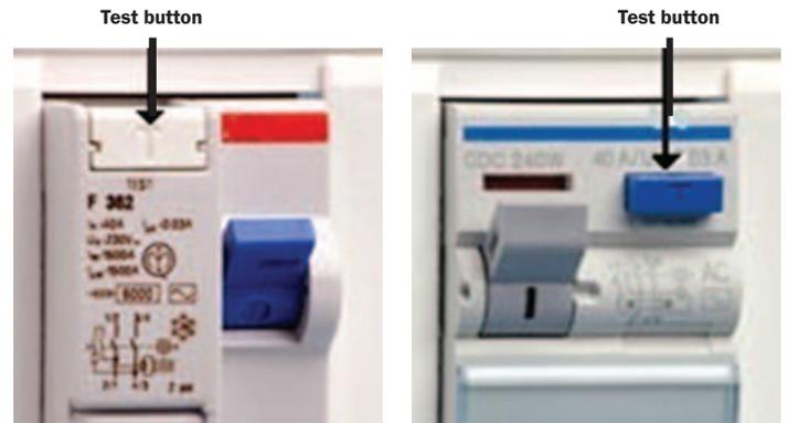
Picture 3: Two different types of Residual Current Devices including the test buttons.
